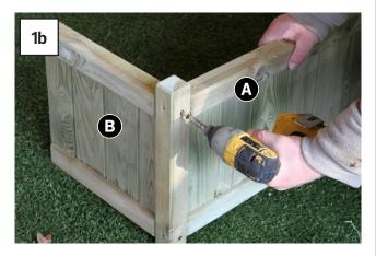
Locate Side Panels (B) into slots in Front Panel (A). Fix in position using 4x 90mm screws.
