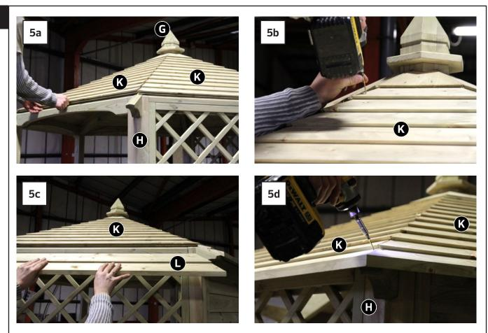
(N.B. Prior to fixing Roof Panels, apply two even beads of silicone to each Rafter D and into grooves in Finial G.)
