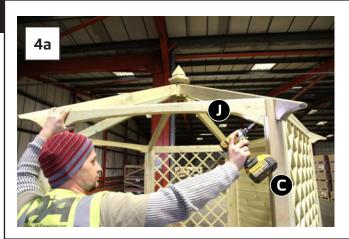
Fix Fascia J between Posts C above Balustrade Panels F and entrance using 6no 70mm screws (2no per Fascia) – Fig.4.
