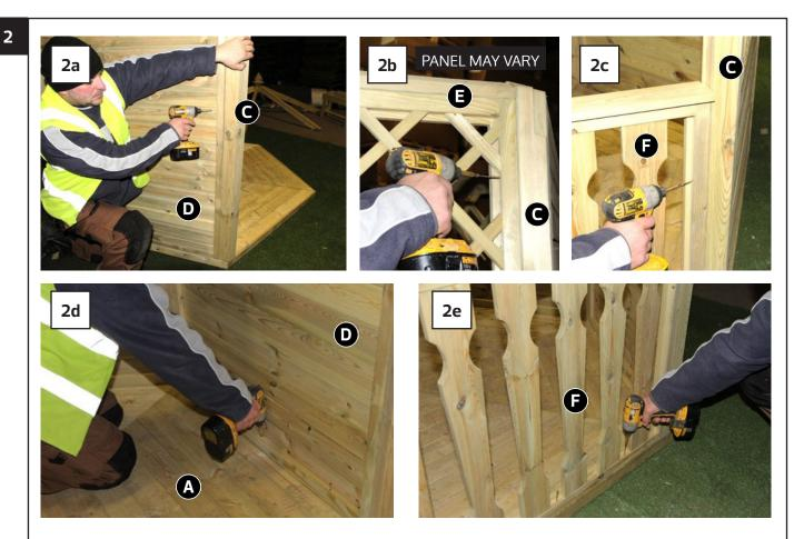
Attach 2no Posts C to Full Panel D using 6no 70mm Screws (3no per post) as shown in Fig.2a. Further attach 2no Trellis Panels E to Posts C using 6no 70mm Screws (3no per post) to form the back wall of Gazebo (Fig.2b).
