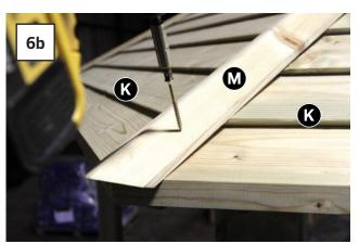
Apply Expansion Tape to underside of Roof Capping M (Fig.6a), position over roof panel joint and fix using 6no 45mm Screws (3no per side) - Fig.6b. Repeat procedure for remaining 5no Roof Cappings M.
