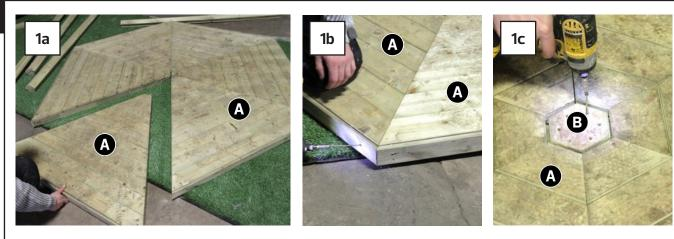
Lay out 6 Floor Panels A as shown in Fig.1a and fix together using 12no 70mm Screws as shown in Fig.1b. Place the Infill B in centre and fix in position using 6no 45mm Screws (Fig.1c).
