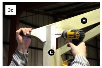
Insert 6no Rafters H into predrilled holes of Finial G (Fig.3a) and fix in position using 6no 120mm Screws (1no per Rafter H). Lift Rafter Assembly into slots on top of Posts C (Fig.3b) and fix in position using 12no 70mm Screws (2no per post) – Fig.3c.
