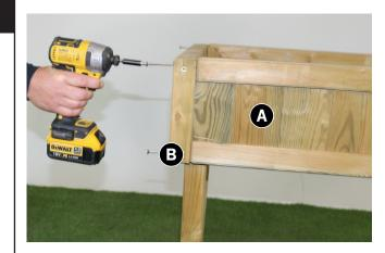
Insert opposite ends of Side Panels (A) into slots in remaining Leg Assembly (B) and fix using 4 x 80mm Screws (2 x Screws per Side Panel (A)).
