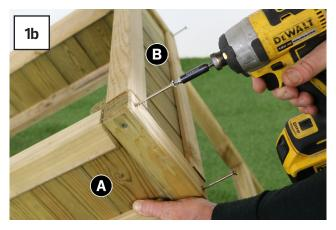
Insert ends of 2 x Side Panels (A) into slots in Leg Assembly (B) and fix using 4 x 80mm Screws (2 x Screws per Side Panel (A)).
