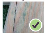
Owing to timber's natural moisture content, variations in temperature and humidity can cause expansion and contraction and may result in cracks and splits in any product made from natural timber. Any cracks and splits in the timber grain will alter with the changing seasons. They do not compromise the strength and durability of the product - they just add to its unique character.
