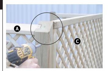
Position Rectangular Trellis Panel (C) to rear posts of Side Panels (A) (flush with back and top of posts) and fix using 4 x 60mm screws (2 x per side).
