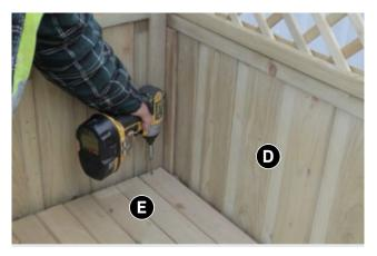
Insert Base Panel (E) and fix using 4 x 40mm screws (1 x Screw per corner).
