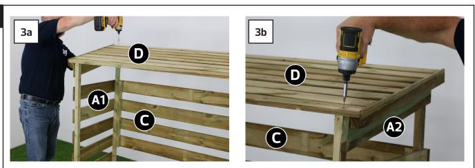
Place Roof Assembly (D) onto Side Panels A1& A2. Before fixing roof to side panel measure and leave 15mm overlap to the back of the log store. Place 1x 4x50mm screw in each corner ensuring it is fixed to the Side Panel A1& A2 Top Frame as per image.
