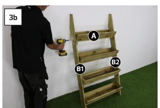
Set out Side Rails B1 & B2 as shown in Fig. 1a. Place 1x Trough (A) onto lowest battens making the trough flush with the back of the side rail and fix using 4x 60mm screws (2x 60mm screws at each end, pre drilling them first).
