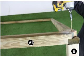
Position 2 x Posts (B) beneath Ring Beam (A1) and attach using 2 x 120mm Screws, (1 x 120mm screw per post.).
