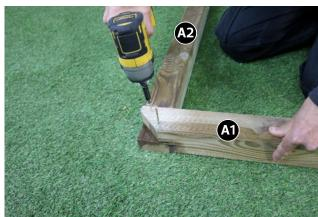
Set out Ring Beams A1 & A2 as shown above and fix in position using 8 x 60mm screws, (2 x 60mm Screws per corner.).
