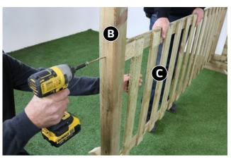
Position 1 x Hand Rail (C) between Posts (B) at desired height and fix using 4 x 120mm Screws, (2 x 120mm per post.), Repeat for remaining 2 x Hand Rails (C)
