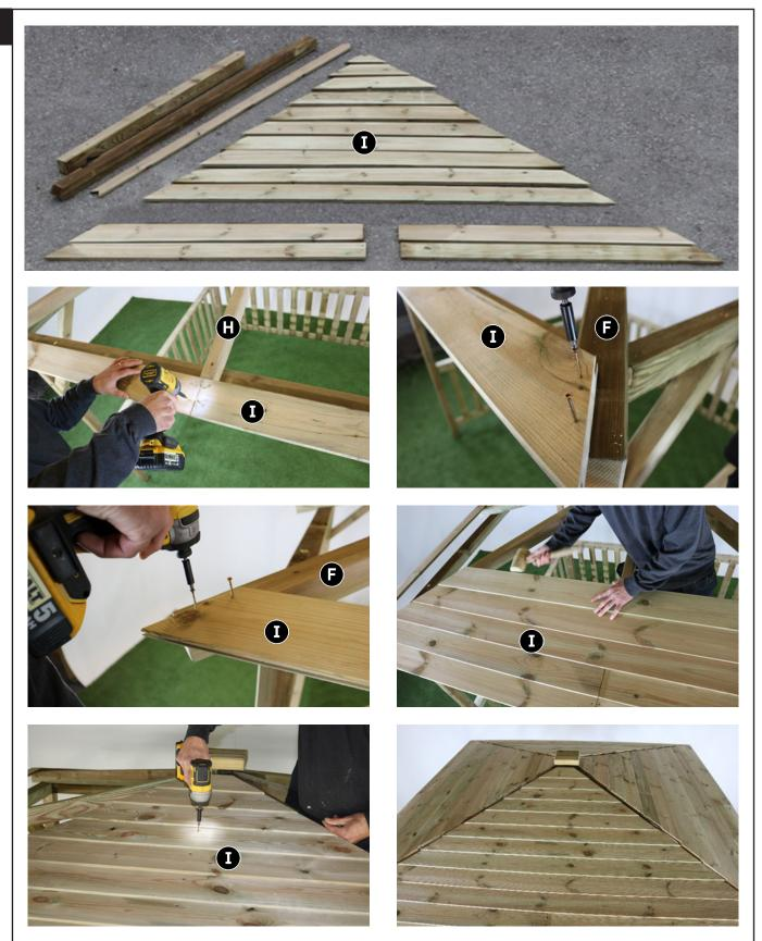
Open 1 x Roof Board pack and set out as shown above (Top). Attach longest pair of square ended roof boards to Centre Rafter (H) and to Rafters (F) (allowing a 10–15mm overlap beyond rafter ends) using 8 x 45mm Screws. (4 x 45mm Screws per board, 2 x 45mm Screws per end).
