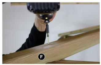
Attach remaining 2 x Rafters (F) to Finial Block (G) using 2 x 100mm Screws, (1 x 100mm Screw per Rafter (F)), and to Ring beam using 2 x 100mm Screws (1 x 100mm screw per Rafter (G)).
