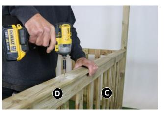
Place 1x Handrail Cover (D) onto Handrail (C) and fix using 4 x 45mm Screws. Repeat for remaining 2 x Handrail Covers (D) and Handrails (C)
