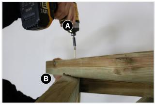
Place rafter assembly diagonally onto ring beam and fix using 2 x 100mm Screws, (1 x 100mm Screw per rafter.).
