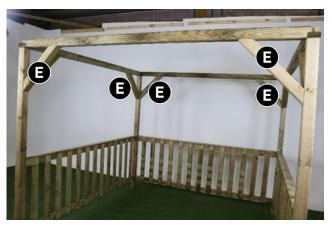
Fix 1 x Bracing (E) to Post (B) & Ring beam using 2 x 140mm Screws as shown above. Attach remaining Bracings (E) to Posts (B) & Ring beam using 16 x 140mm Screws, 2 x Screws per Bracing, 2 x Bracings per Post.
