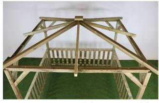
Attach 1x Centre Rafter (H) to Final Block (G) using 1x 100mm Screw and to Ring beam using 1x 100mm Screw.
