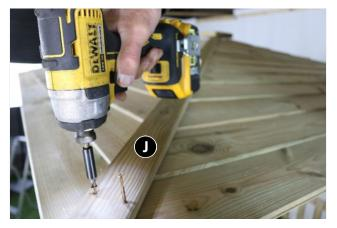
Place 1x Long Cover Strip (J) over joint in roof boards and under finial block capping (angled cut beneath capping and facing upwards). Fix in position using 8 x 45mm screws (2 x 45mm screws per end, 2 x 45mm either side of centre).
