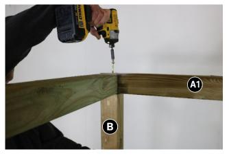
Place remaining Posts (B) beneath Ring Beam and fix using 2 x 120mm Screws, (1 x 120mm screw per post.).
