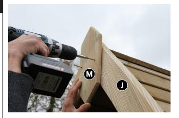
Position and attach centrally, 2 x Pointed Finials M to the Fascia Boards J (front and back) using 4 x 40mm screws – 2 x per finial (Fig.10)
