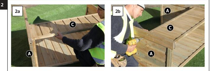
Place Front Panel (C) between the Side Panels (A) (Fig.2a) and fix in position using  $4 \times 60$ mm Screws – 2 per side (Fig.2b).
