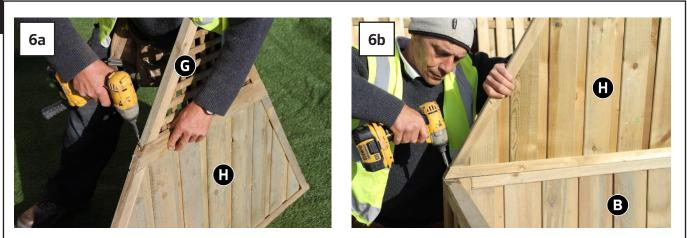
Attach Trellis Back Panel G to the Middle Back Panel H using 2 x 40mm Screws – 1per side (Fig.6a). Attach trellis and middle back panel assembly to the Back Panel B using 3 x 40mm Screws 1per corner and 1 in the middle (Fig.6b).
