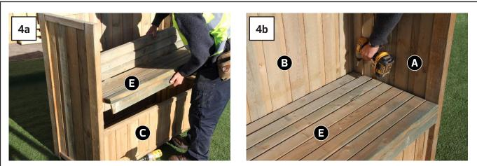
Position the Seas Hinged Assembly E on to the seat support battens (Fig.4a) and fix to the seat support battens using  $4 \times 60$ mm Screws – 2 per side of rear section of the Hinged Seat Assembly E (Fig.4b).
