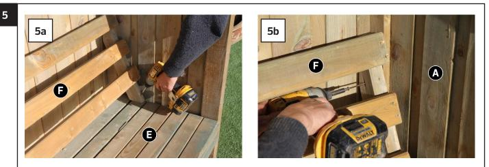
Position Seat Back Rest F between the Side Panels A (Fig.5a). Attach to the Hinged Seat Assembly E using 2 x 60mm Screws – 1 per side (Fig.5a) and to the Side Panels A using 2 x 60mm Screws 1 per side (Fig.5b)
