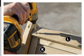
Attach the Ridge Capping L to the top of Roof Panels K using 6no 40mm Screws – 3 x per panel (Fig.9).
