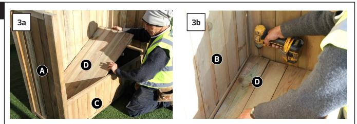
Locate Floor Panel D on to the floor support battens (Fig.3a) and fix to the floor battens using 4 x 60mm Screws – 2 per side.
