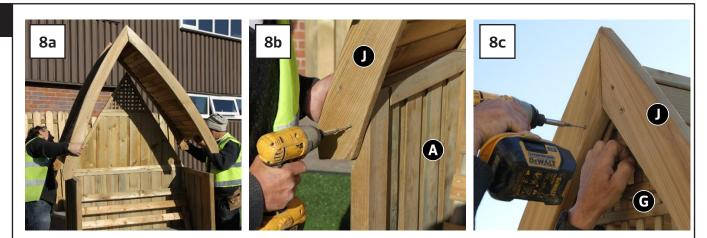
Place roof assembly on to Side Panels A (Fig.8a) and fix to the Side Panels A through Fascia Boards J using 4 x 60mm Screws – 1 per Fascia Board. Further attach the roof assembly to the Trellis Back Panel G through the Fascia Boards J using 2 x 50mm Screws – 1no per rear Fascia Board J.
