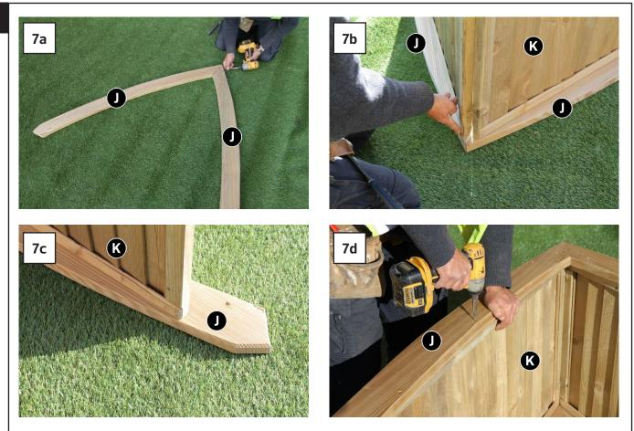
Fix together 2 x Fascia Boards J using 1 x 60mm Screw. Repeat process for the remaining 2 Fascia Boards J. Set the Roof Panels K as shown in Figs. 7b & 7c ensuring the outermost corners of the Roof Panels K are flush to the top edges of Fascia Boards J (Figs.7b & 7c). Attach Fascia Boards J to Roof Panels K using 12 x 50mm Screws – 3 per Fascia Board J (Fig.7d).
