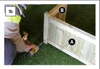
Locate Side Panels (B) into slots in Front Panel (A). Fix in position using 4no 90mm screws. See Figs 1a & 1b.
