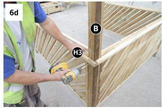
Attach Shelf Support Battens (Med.) internally to left and right hand posts using 4x 60mm screws (2 per batten). (See Fig. 6a)
