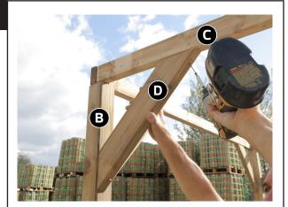
Fix 8x Bracings D to posts and ring beam assembly using 16x 60mm screws (2 per bracing). (See Fig. 3)
