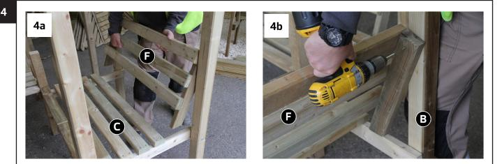
Position Back Rest F onto Seat C (Fig.4a) and fix in position using 4x 60mm Screws – 2x to Seat F (see arrows in Fig.4a) and 2x to posts (Fig.4b). Repeat procedure for remaining Back Rest F.
