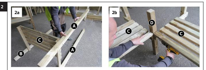
Attach 2x Notched Posts A and 1x Full Post B to remaining seat C (ensuring notches facing outwards) using 3x Bolts, Washers & Nuts –1x per post. See Fig.2a. Attach seat and posts assembly to Table Leg D using 2x 60mm Screws –Fig.2b
