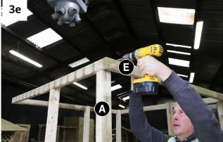
Locate Ring Beam E into notches of Notched Posts A (right side front facing the arbour), flush with Notched Post A as shown in Fig.3a. Using Side Panel J to set the distance between Notched Posts A, fix Ring Beam E in position using 4x 60mm Screws –2x per post.
