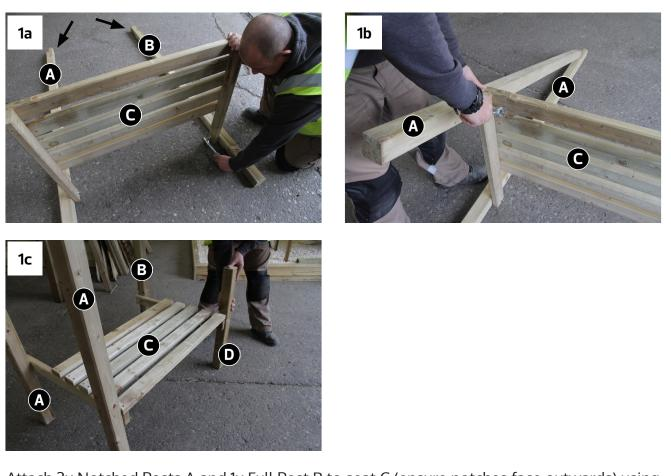
Attach 2x Notched Posts A and 1x Full Post B to seat C (ensure notches face outwards) using 3x Bolts, Washers & Nuts –1x per post. See Fig.1a & 1b. Further attach Table Leg D to Seat C using 1x Bolt, Washer & Nut –See Fig.1c
