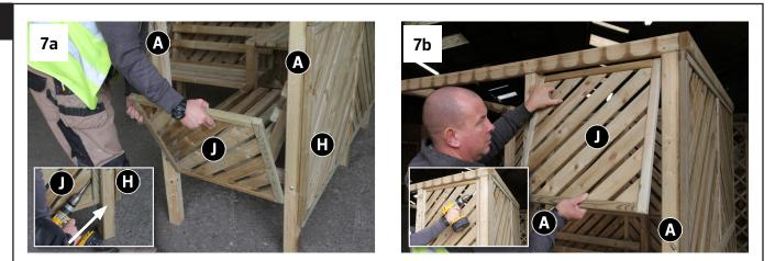
Locate 2x Side Panels J between Notched Posts A (ensure top Side Panel J meets underside of Ring Beam E and bottom Side Panel J is in line with the underside of Back Panel H) as shown in Fig.7a & 7b. Fix in position using 8x 60mm Screw –4x per Side Panel J. Repeat procedure for remaining Side Panels J.
