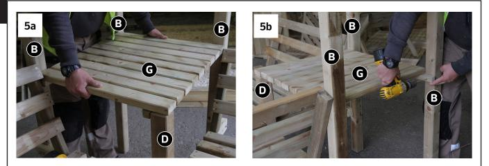
Position Table Top G onto Table Leg D and between Full Posts B as shown in Fig.5a. Ensuring Table TopG is levelled, fix in position through Table Top G battens using 4x 60mm Screws – 1x into each Full PostB & 1x into Table Leg D. See Fig.5b.
