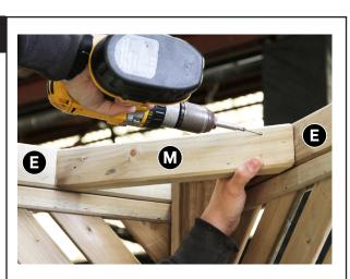
Attach Rear Corner Brace to Ring Beams E as shown in Fig.10 using 4x 60mm Screws –2x per side.
