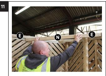
Attach Centre Brace N to Ring Beams E as shown in Fig.11 using 4x 60mm Screws –2x per side.
