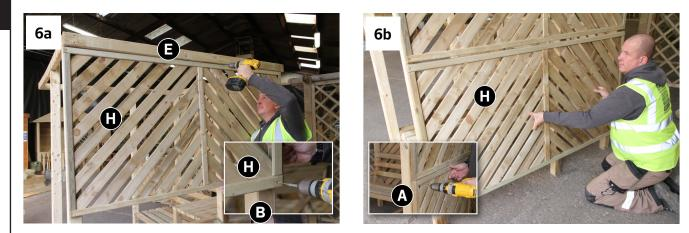
Attach 2x Back Panels H to posts to rear of seat assembly (ensure top Back Panel H meets the underside of Ring Beam E) as shown in Fig.6a and 6b using 12x 60mm screws –6x per panel. Repeat procedure for remaining Back Panels H.
