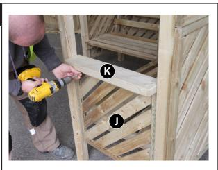
Attach Arm Rest K to Side Panel J as shown in Fig.8 using 2x 60mm Screws. Repeat procedure for remaining Arm Rest K.
