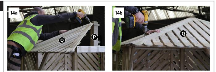
Position Roof Panel Q onto Finial P and Ring Beam E and attach to Finial P using 1x 60mm Screw as shown in Fig.14a. Repeat procedure for remaining Roof Panels Q. Ensuring Roof Panels Q are correctly aligned, fix to Ring Beams E using 12x 60mm Screws –3x per Roof panel Q –Fig.14b. Ensuring Roof Panels Q are correctly aligned, fix to Ring Beams E using 12x 60mm Screws – 3x per. Roof panel Q – Fig.14b.
