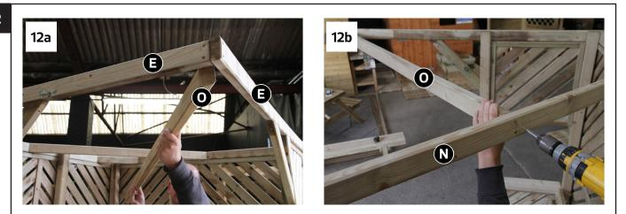
Locate Finial Support O between front Ring Beams corner and middle of Centre Brace N (Fig12a). Fix in position using 4x 60mm Screws as shown in Figs.12a and 12b.
